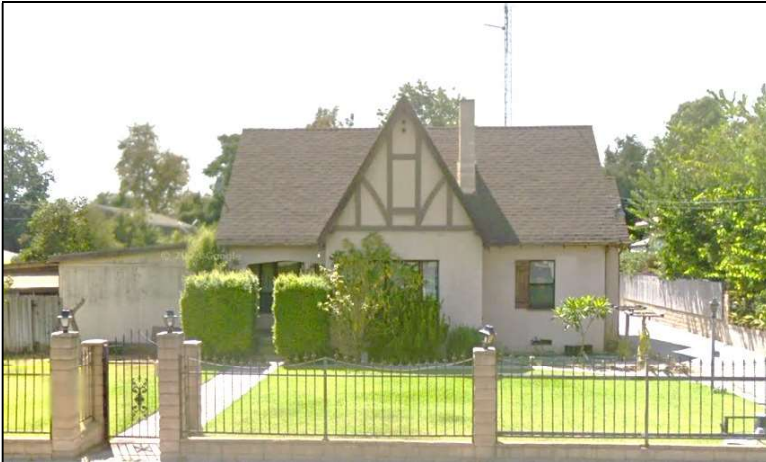
1405 S. 8 th Avenue, view west (Google street view 2012). Shed roof addition is clearly visible at the south end of the façade. There is no window in the gable peak.
